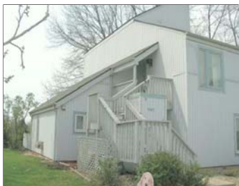
53455 STONERIDGE UNIT B
